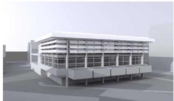
Figure 8: Reflective wings. Highly reflective, diffuse coating on fabric.
