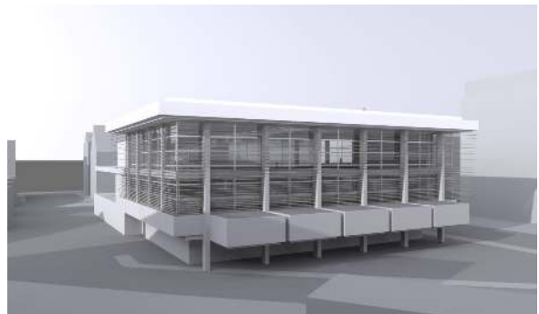
Figure 6: Fixed, tilted external blinds. Big horizontal light shelf on the inside.
